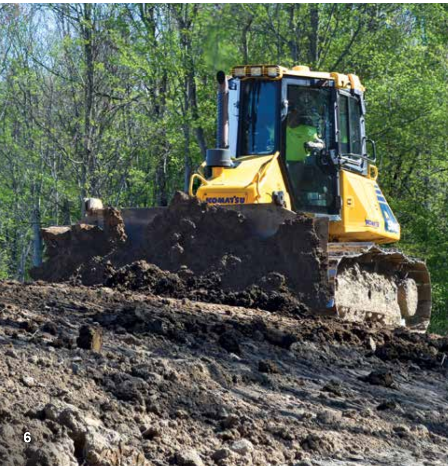
Foreman Will Scarlett grades a bank with a Komatsu D51PXi IMC dozer.
