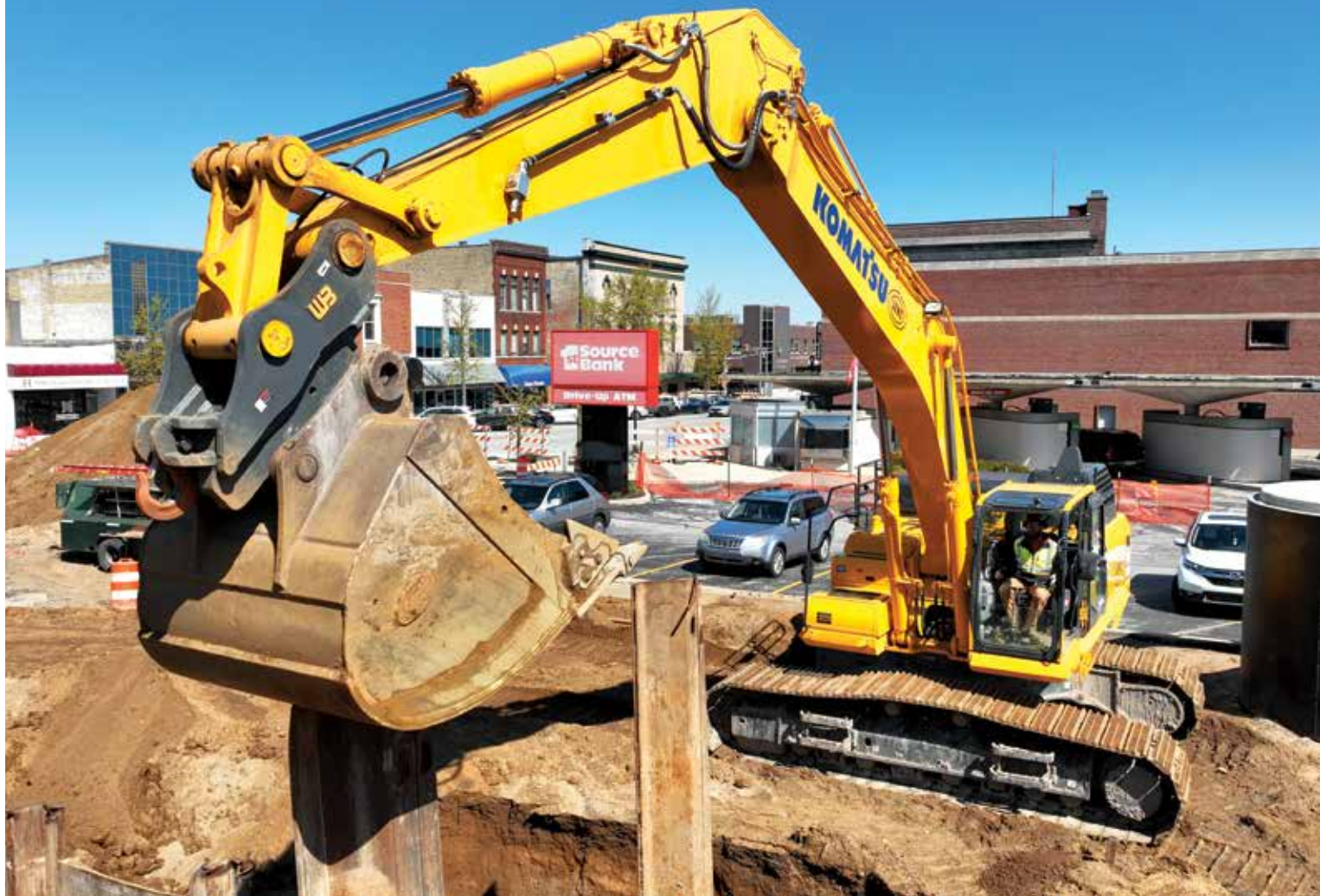
With a Komatsu PC490LC-11 excavator, an operator piles a beam.
