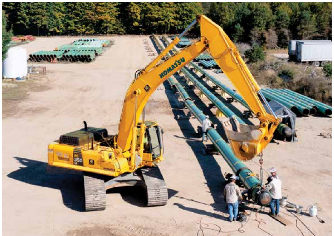
At R.L. Morris & Sons Construction Company's (RLM) pipe yard, an operator lifts a pipe using a Komatsu PC350LC excavator while a crew places the pipe.
