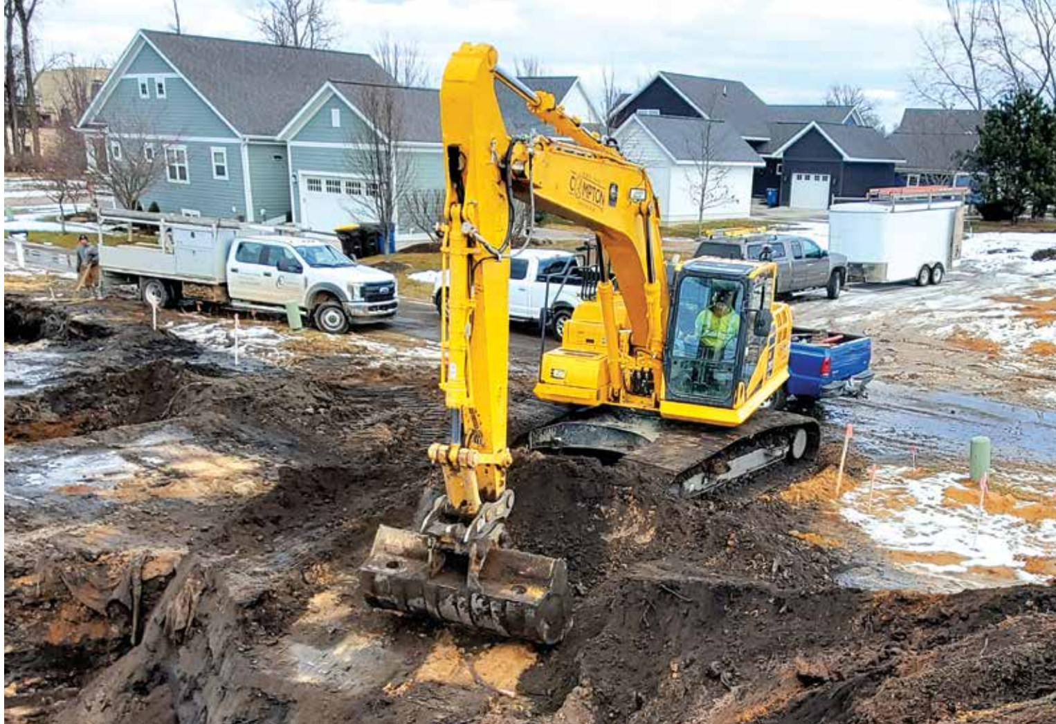
An operator shapes the side of a ditch using a Komatsu PC210LCi-11 excavator. "The GPS excavator has become an indispensable piece of equipment for us," noted Marc Compton, owner of Compton Inc. "The grade control on the excavator has given us a lot of confidence."
