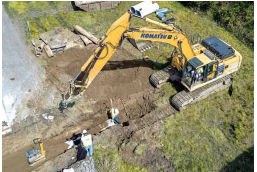
This crew from Malley Construction uses a Komatsu PC360LC excavator to install a cross culvert.
